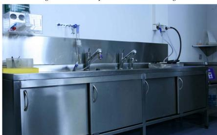
Figure 13-3: Sink required for manual cleaning
